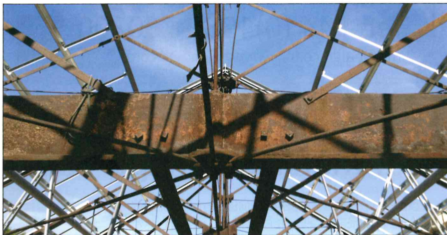
The foundry, designed by John Urpeth Rastrick in 1820, was at the time considered a state-of-the art building due to its pioneering use of 50 foot-long cast iron beams, with wrought iron tie bars running north-south, east-west, and diagonally, throughout, as a supporting framework for its roof.
